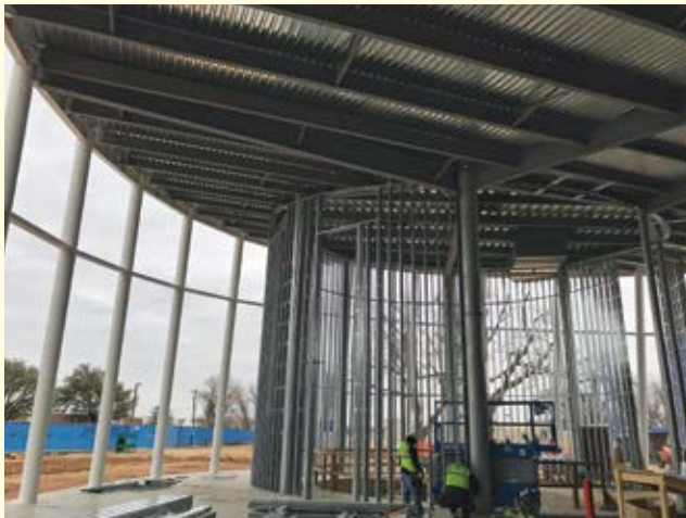
The planetarium's interior walls under construction
