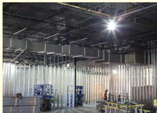
Interior wall framing under way
