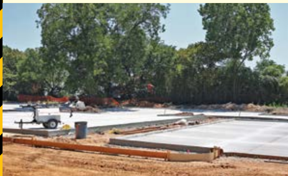
The southeast parking lot surface nearing completion
