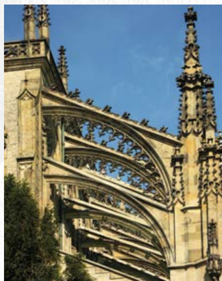
Figure 5. Flying buttresses employed in cathedral construction are remarkably efficient and serve a specific load-bearing function.
