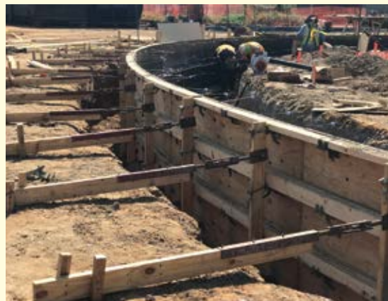
Forms in place for upcoming exterior and slab/foundation
