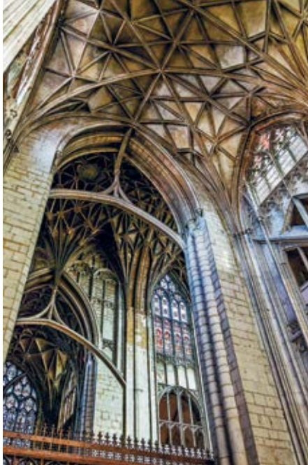
Figure 2. Gloucester Cathedral, Gloucestershire, UK. Defying gravity for centuries, each arched rib in the vaulted ceiling was precisely designed and set in place for efficient support.
