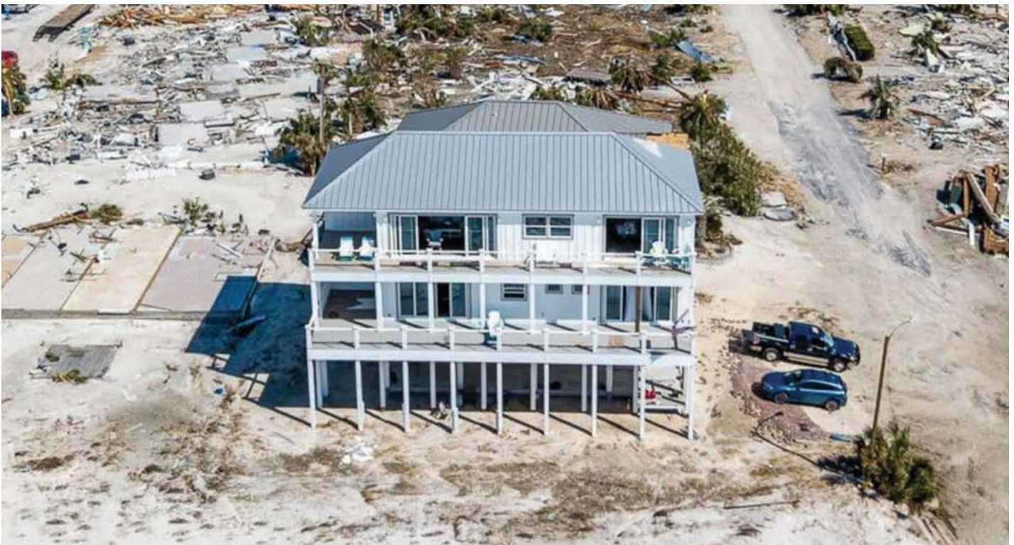
Mexico Beach, Florida, home built by Dr. Lebron Lackey with design specifications for materials and construction methods to withstand 250 mph winds. Did it survive in October 2018 because Hurricane Michael “selected for” one home and “selected against” the others? Of
