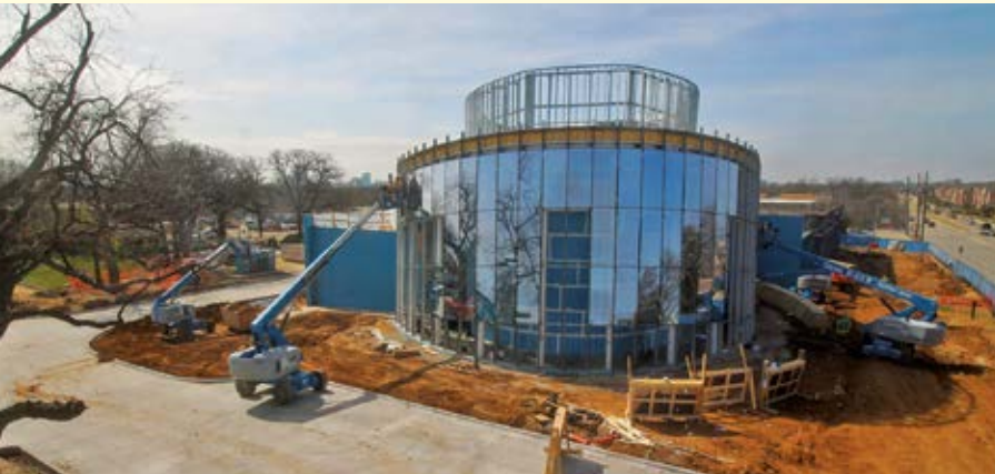
The planetarium's exterior windows are set in place.
