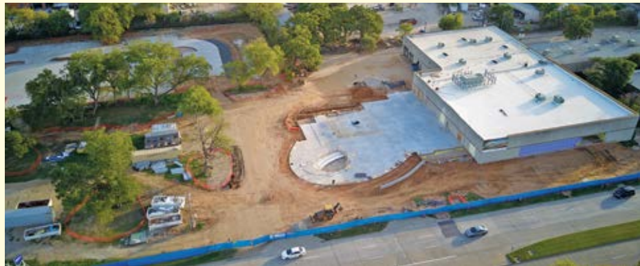
A drone shot of the construction site. Image credit: Parker Eng.
