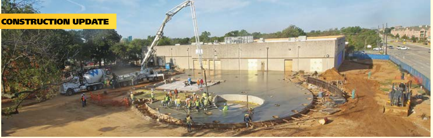
Beck construction crew pours 100s of yards of concrete on October 11, 2017.
