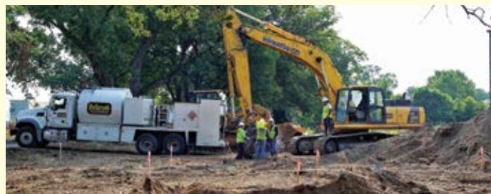
Construction team completes trenching work for property drainage.
