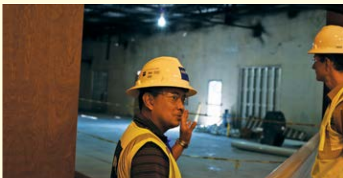
Beck supervisor Paul Palerchio gives an overview of the interior work, including demolition, foundation, excavation for utilities and the Grand Canyon exhibit, location of specific exhibits and the ceiling paint project (painting it black).
