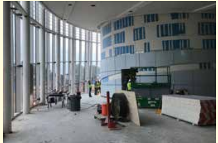
Workers finish the discovery center lobby.
