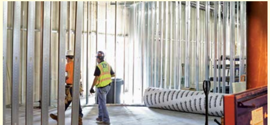
Steel studs in place for the exhibit walls.
