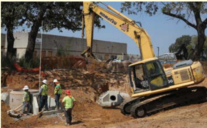
Installing drain heads near the back parking area.
